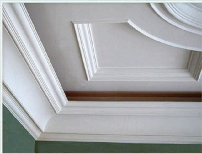
Close-up of sample - Cornice joint installation.
