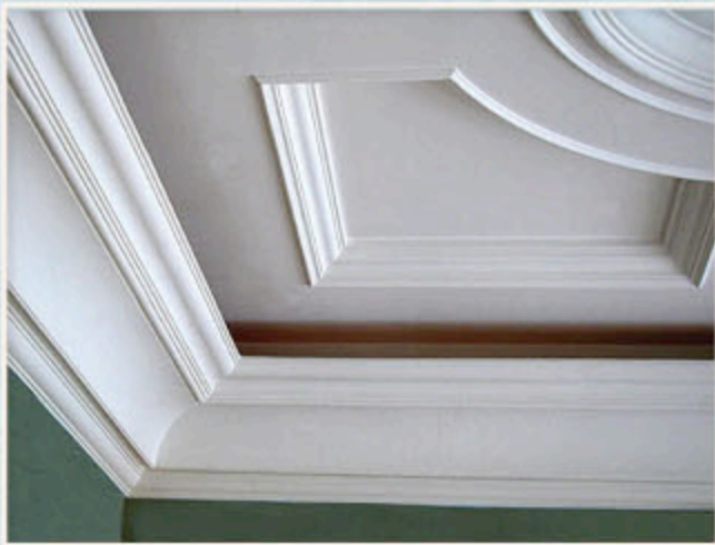
Close-up of sample - Cornice joint installation.
